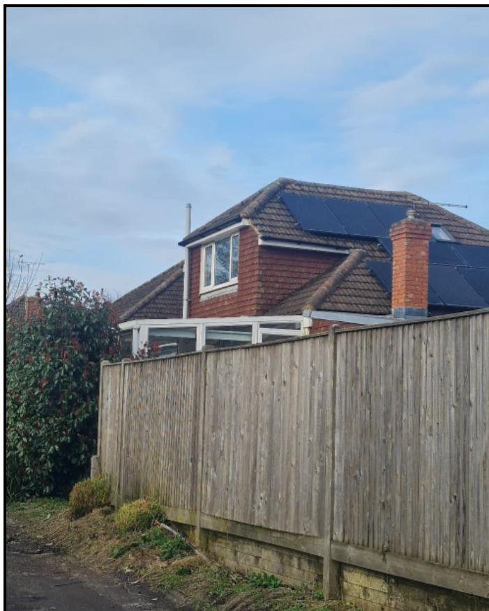
Figure 10 Rear of No 6 Craythorne Facing rear Access Lane
